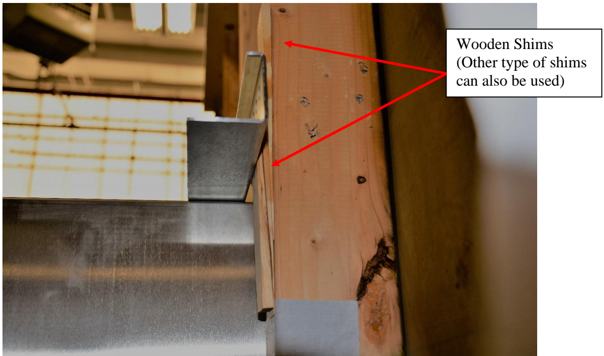
Shims Between Bracket and Wall
