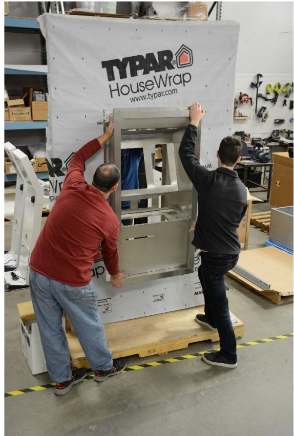
2. Kiosk Assembly Being Pushed into Wall
