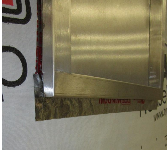
Ice & Water shield Placed Under Metal Edges
