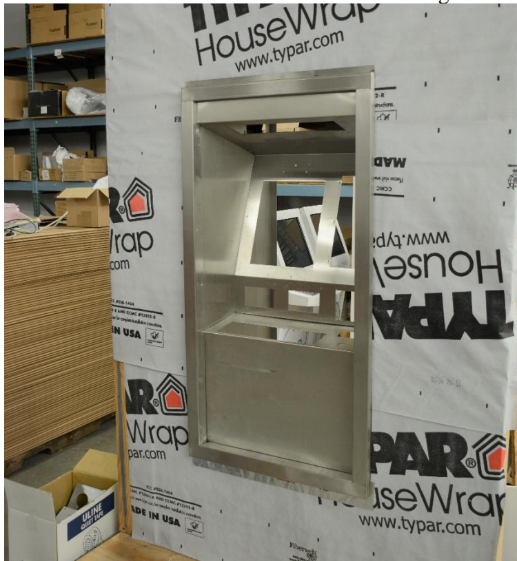
Kiosk Fully Pushed into Wall
